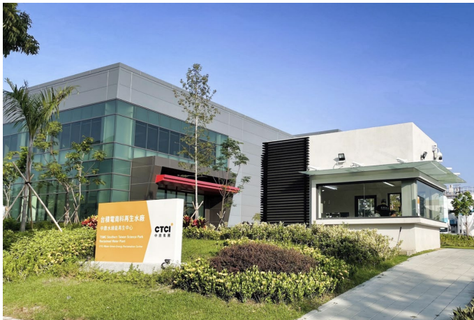
TSMC 's first private water reclamation plant
